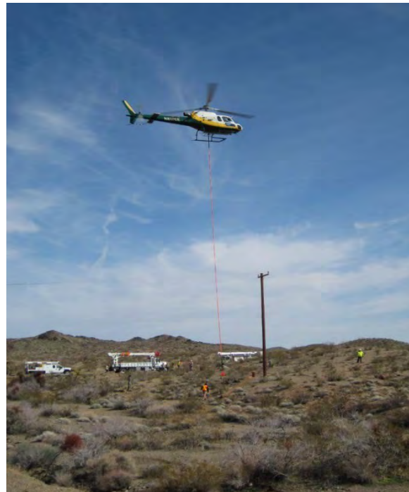
Photo B-15. Pole Set by Helicopter
