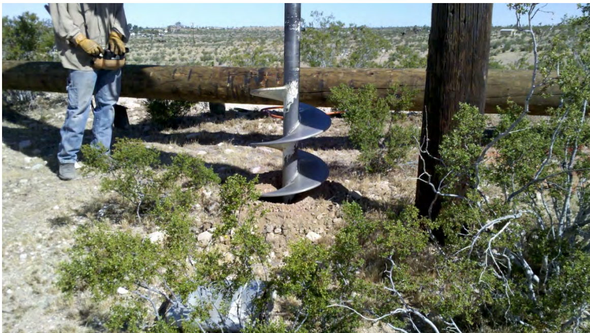
Photo B-10. Drilling New Pole Location
