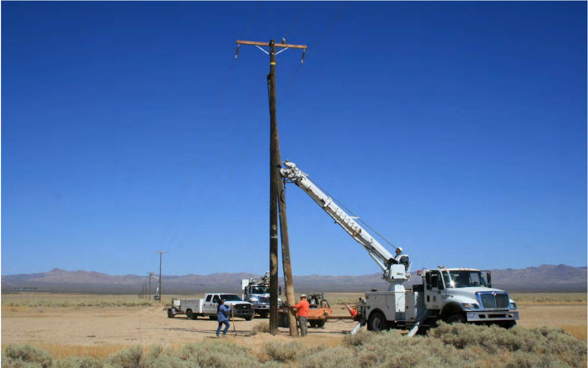
Photo B-13. Use of Line and Boom Truck to Pull Existing Pole from Ground and Place New Pole in Adjacent Hole
