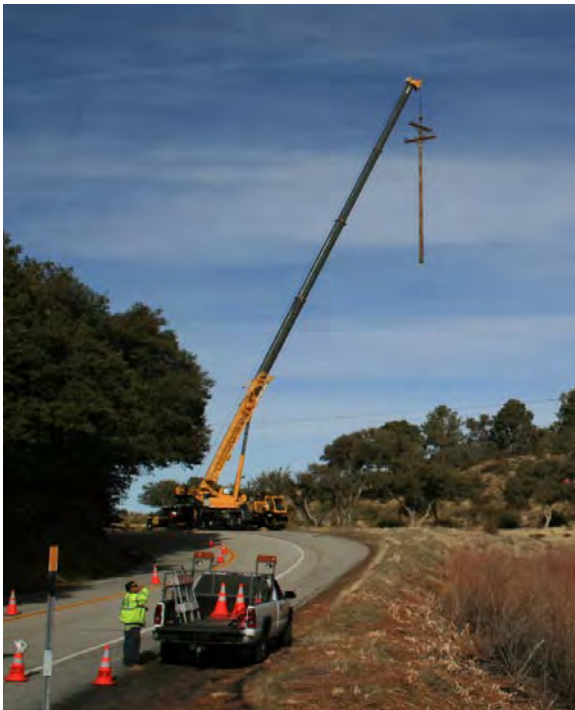
Photo B-14. Pole Set by Crane
