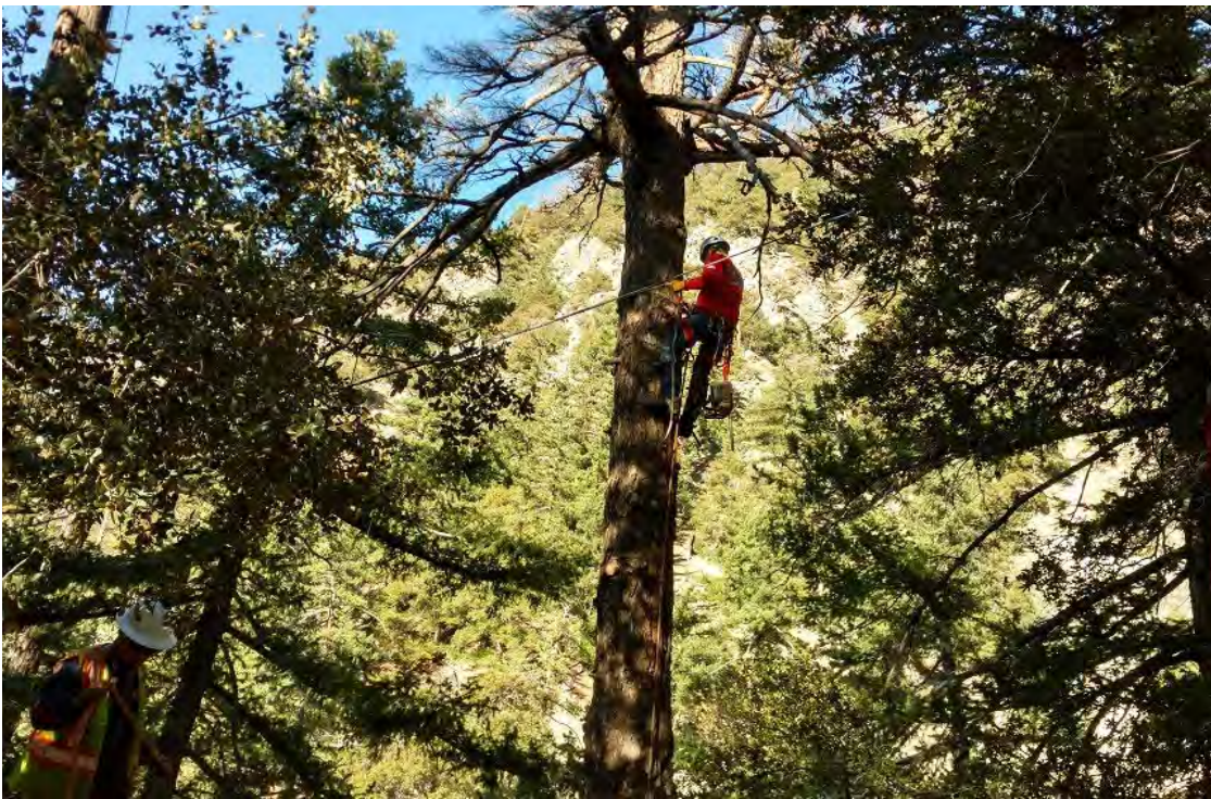
Photo B-17. Utility Crew Topping Hazard Tree
