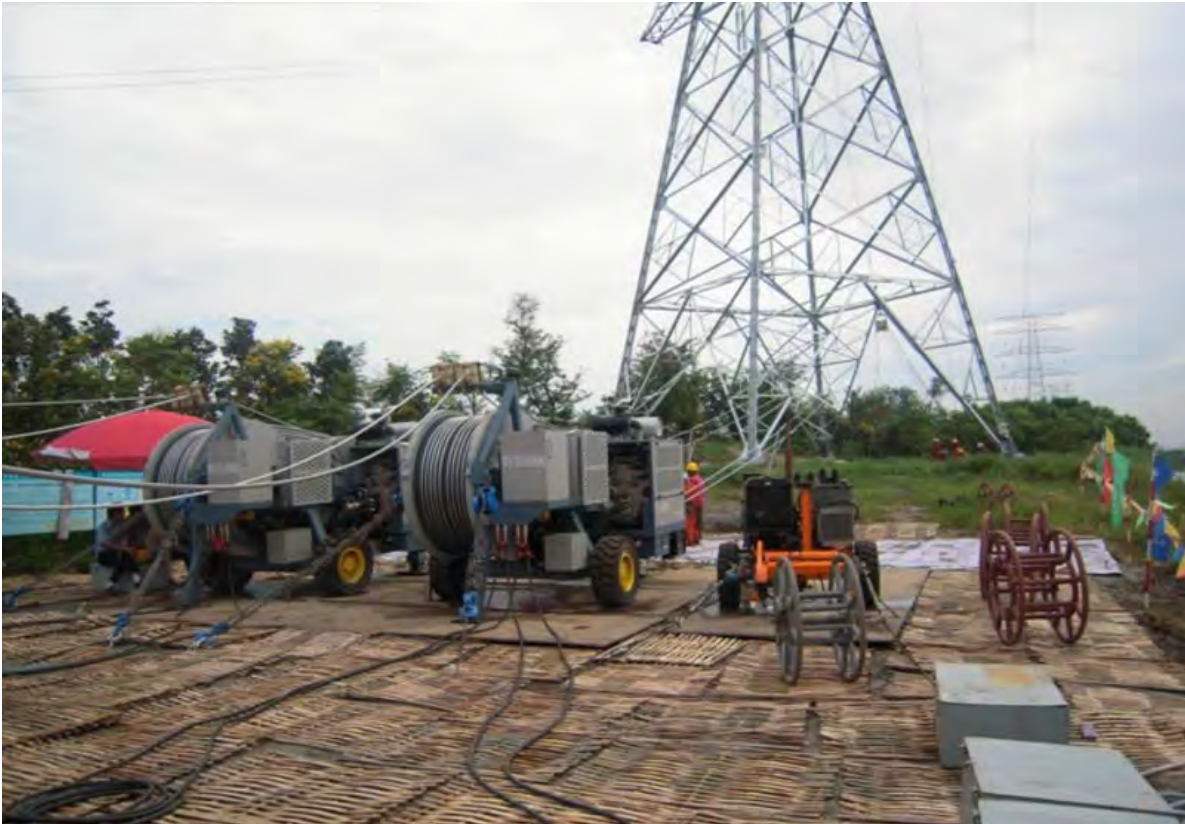
Photo B-18. Example of Large Reconductoring Project
